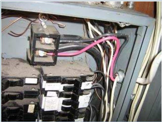
Multi-tapping at bus connectors
