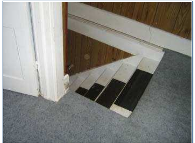
Missing opening guard and hand rail at main stairs
