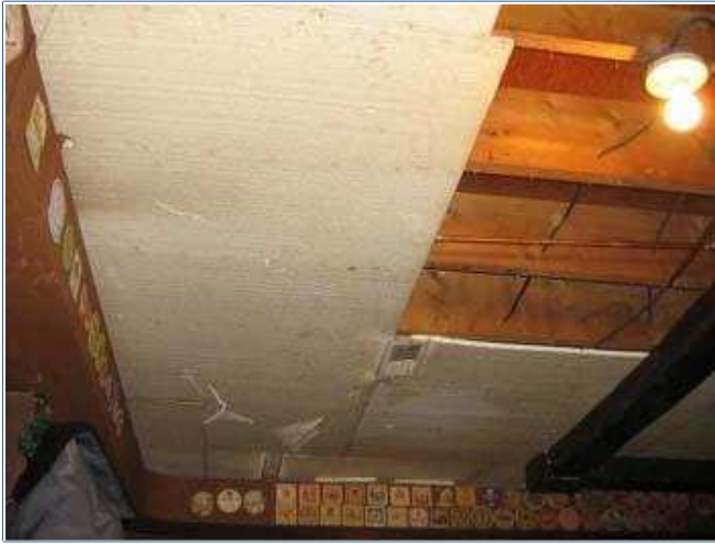
Styrofoam used as ceiling finish material
